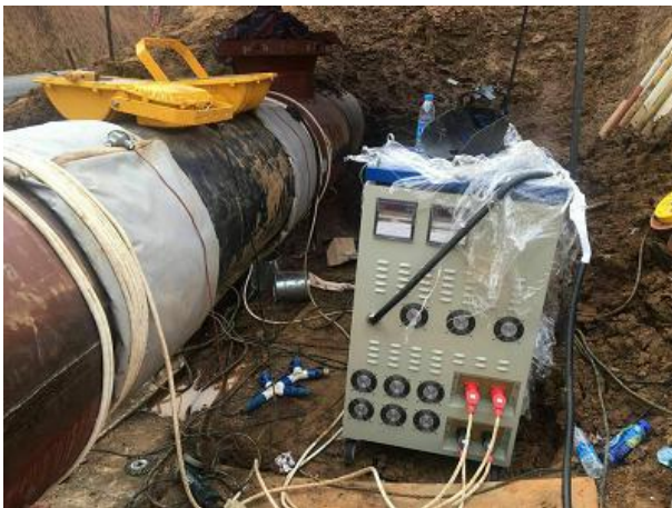
Petroleum Pipeline PWHT
