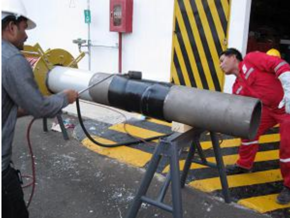
Offshore pipeline coating preheat
