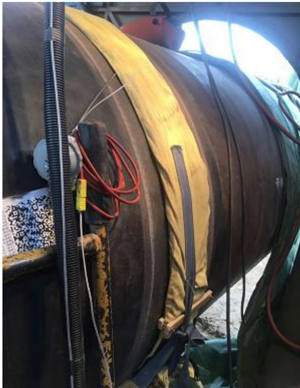
Pipeline weld heating
