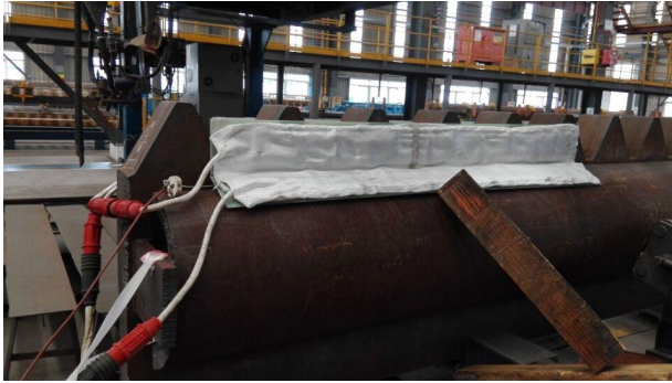
Hydrogen and stress removing after welding of boiler
