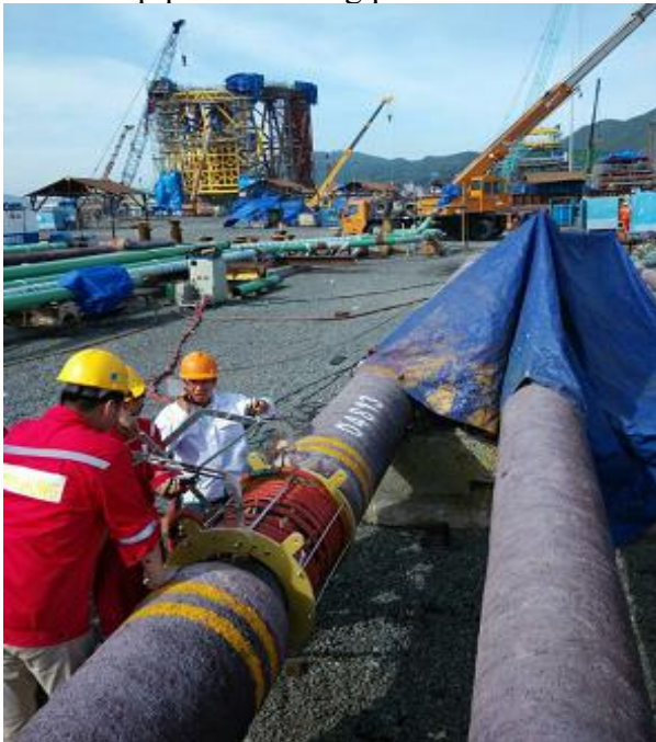
Offshore pipeline coating preheat
